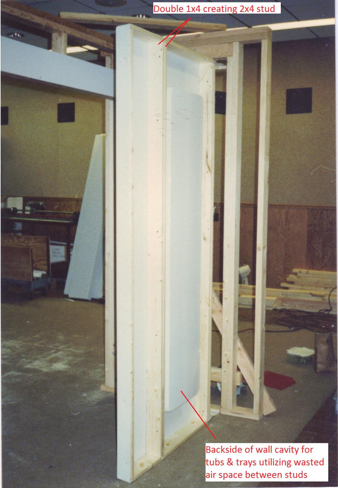
HC shell assembly sandwiched between double 1x4 to create 2x4 studs
