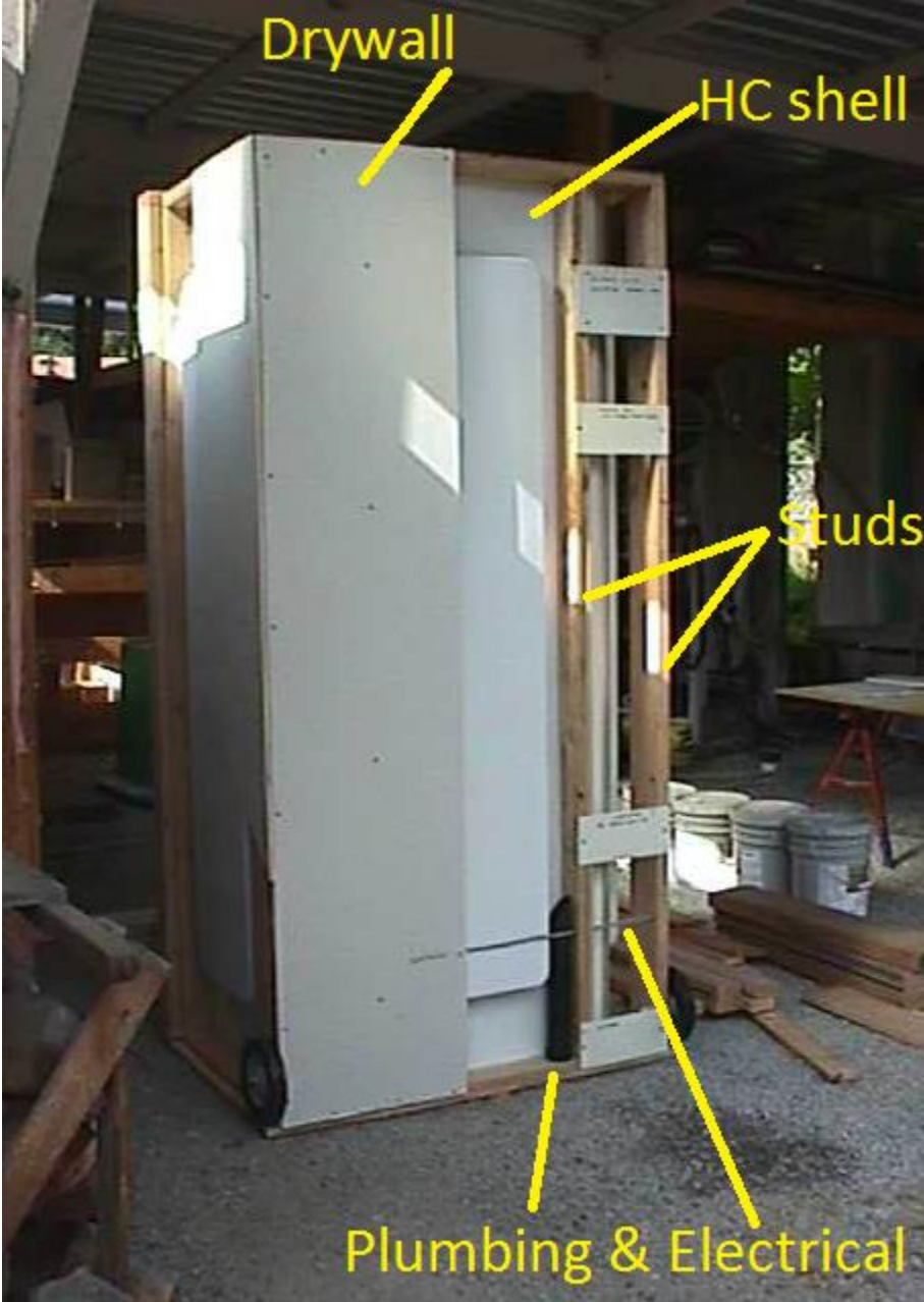
HC backside of model showing drywall, plumbing and electrical
