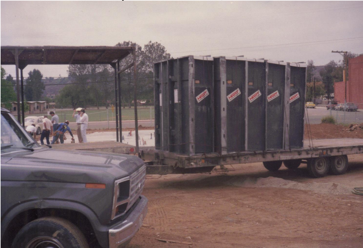
Hart Closets delivered to jobsite. More than 3,000 installed in California.
