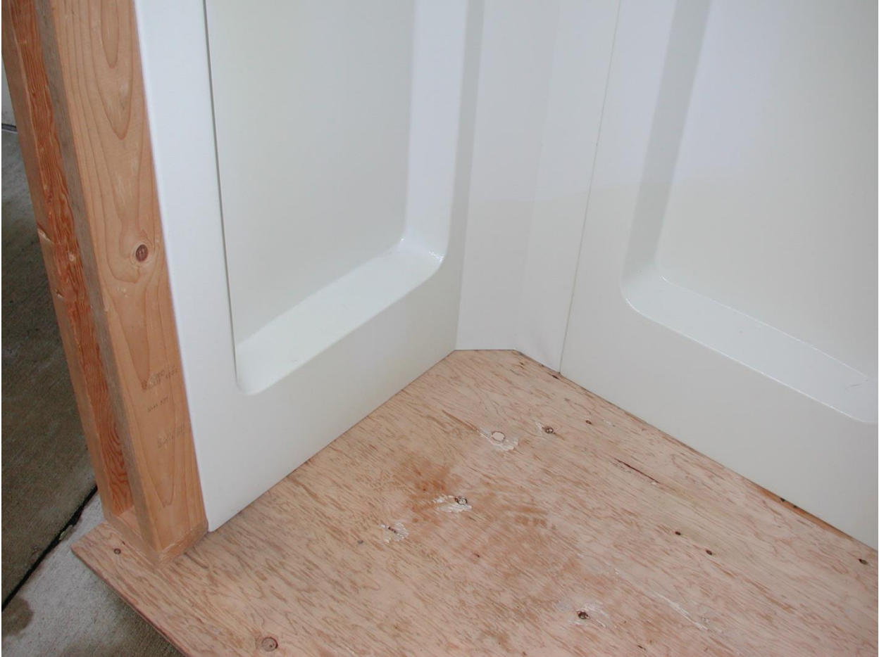
HC fastened to plywood subfloor showing detail
