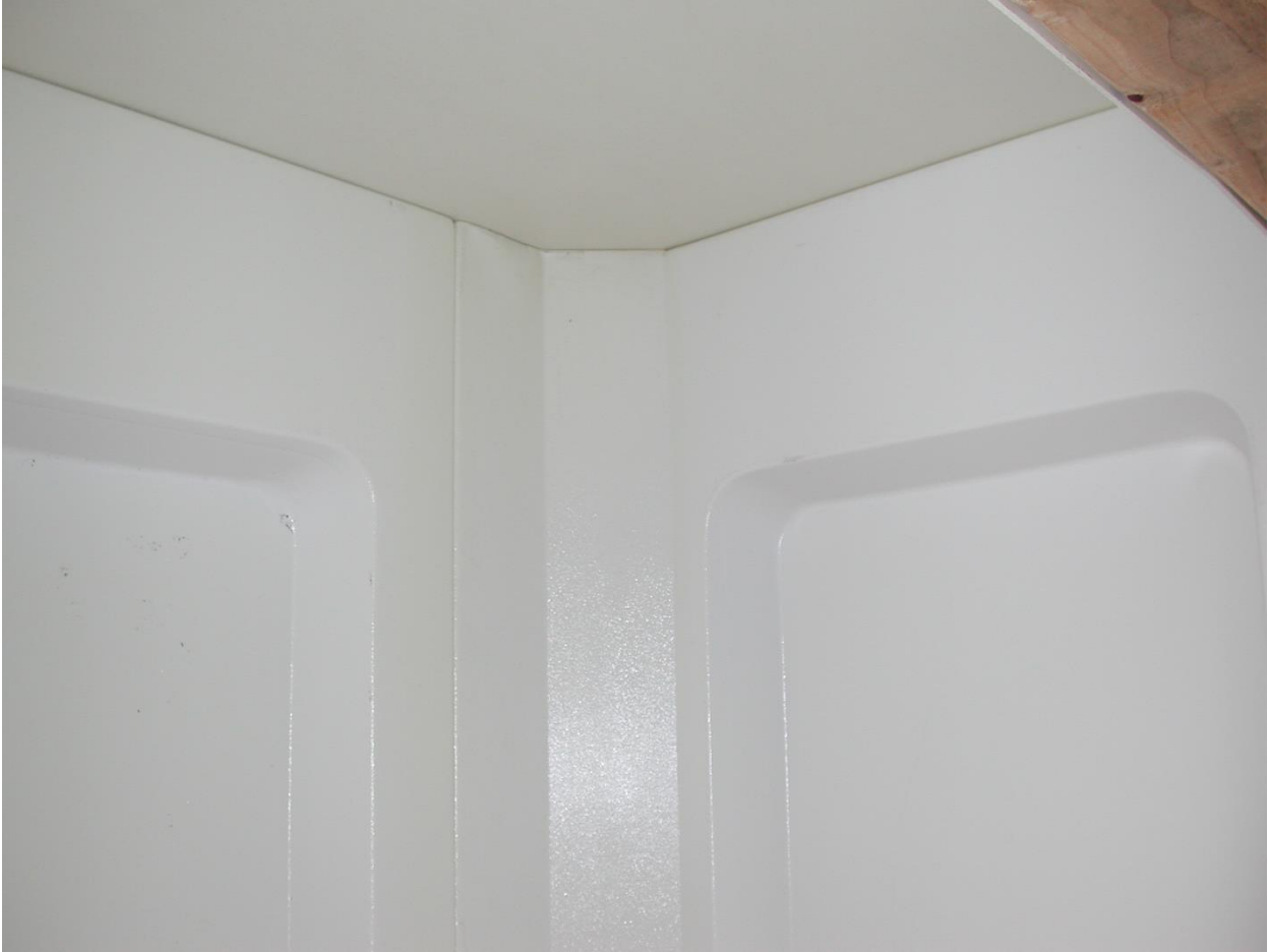
HC ceiling shell assembly
