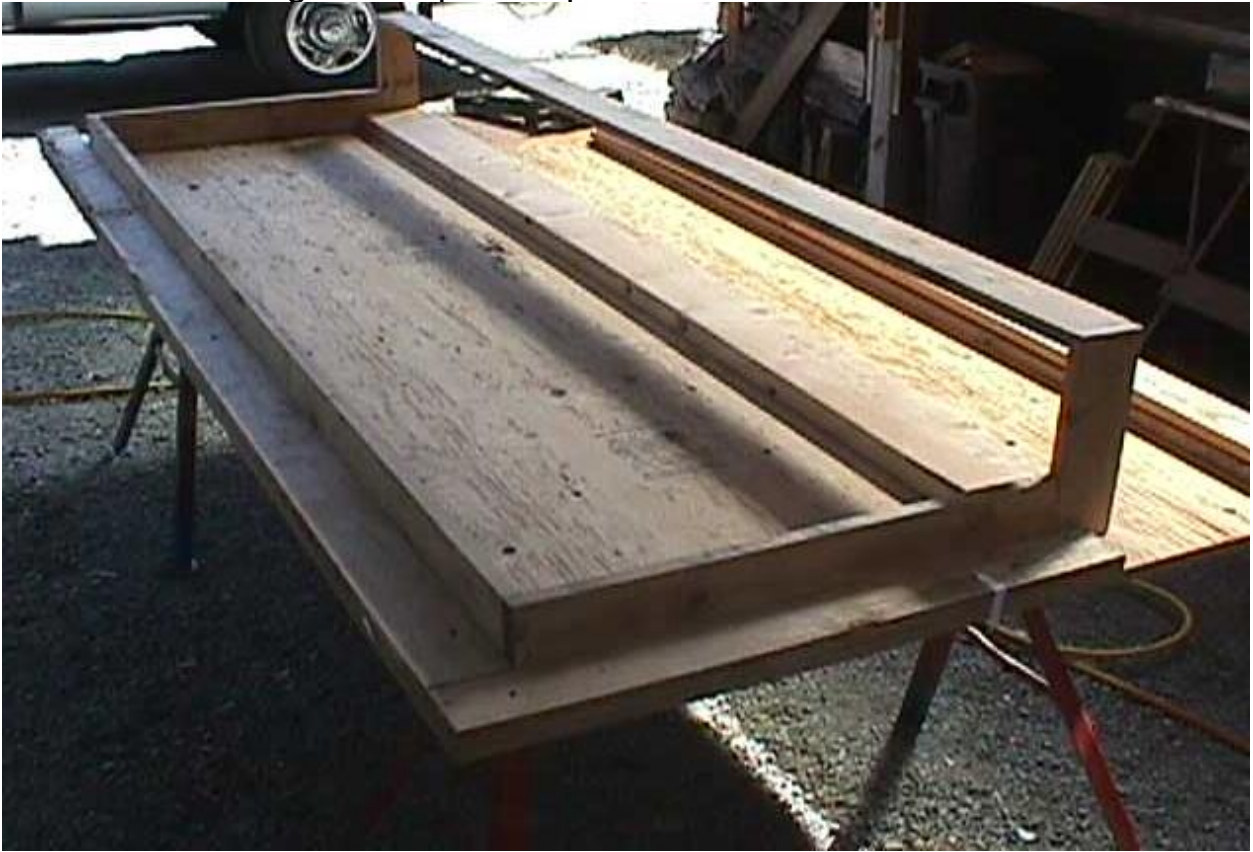
HC corner shell part fastened to framing
