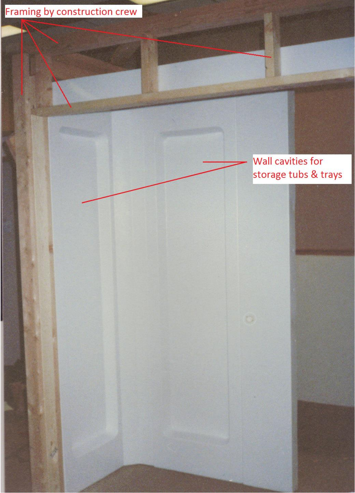
HC shell assembly with wall framing in front
